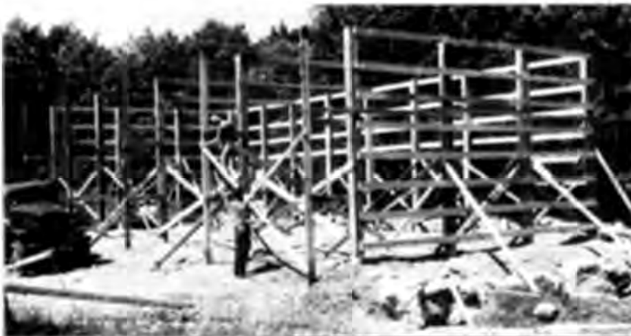
Pole barn construction, July 1988, with timbers from Harvard Forest trees. (Photo by D. Foster)
