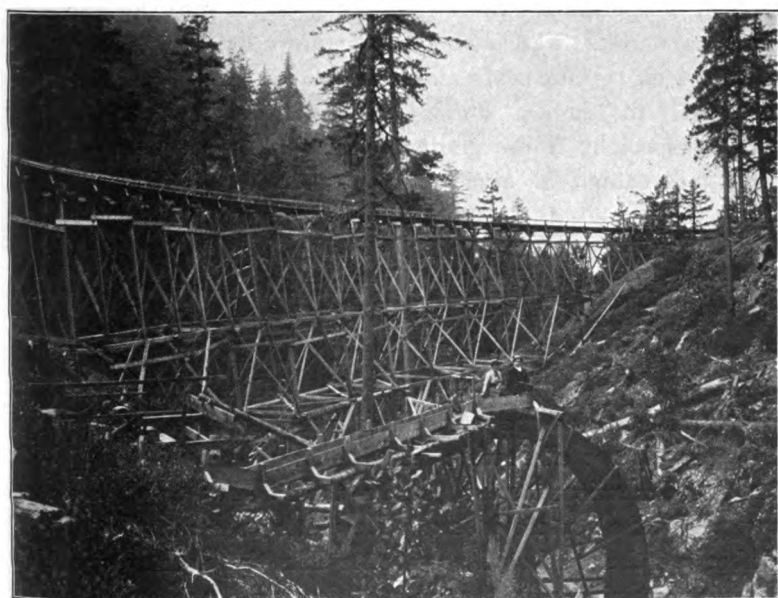
Trestle on a flume in Oregon.
