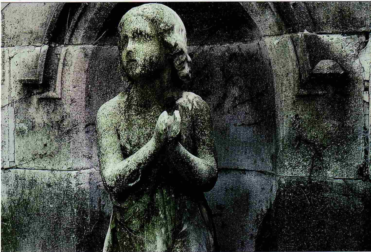
Weathering of this mausoleum sculpture in New York City is hastened by acid rain. Nitric acid and sulfate are the two major components of acid rain; as regulatory controls on sulfur dioxide reduce the amount of sulfate in rain and snow, nitric acid plays an increasing role.
